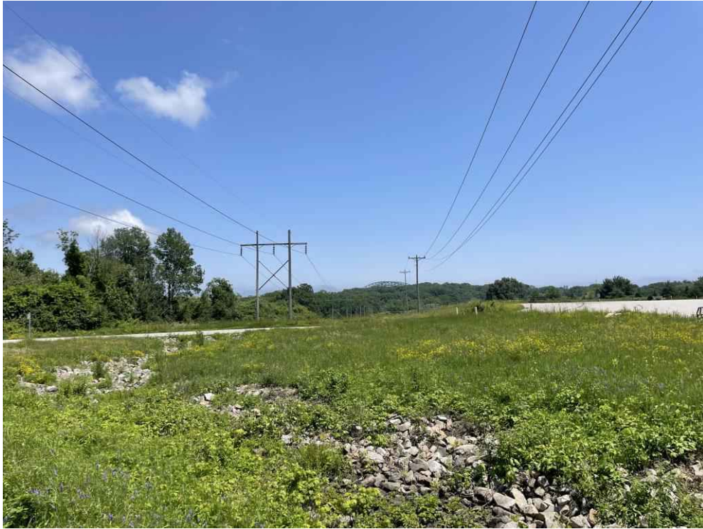
Photograph No. 33: Looking east at Wetland PW-11 (PSS1/PEM1Ex) between Structures 7 and 8 on the T13 Line ROW off Gosling Road, Portsmouth, NH
