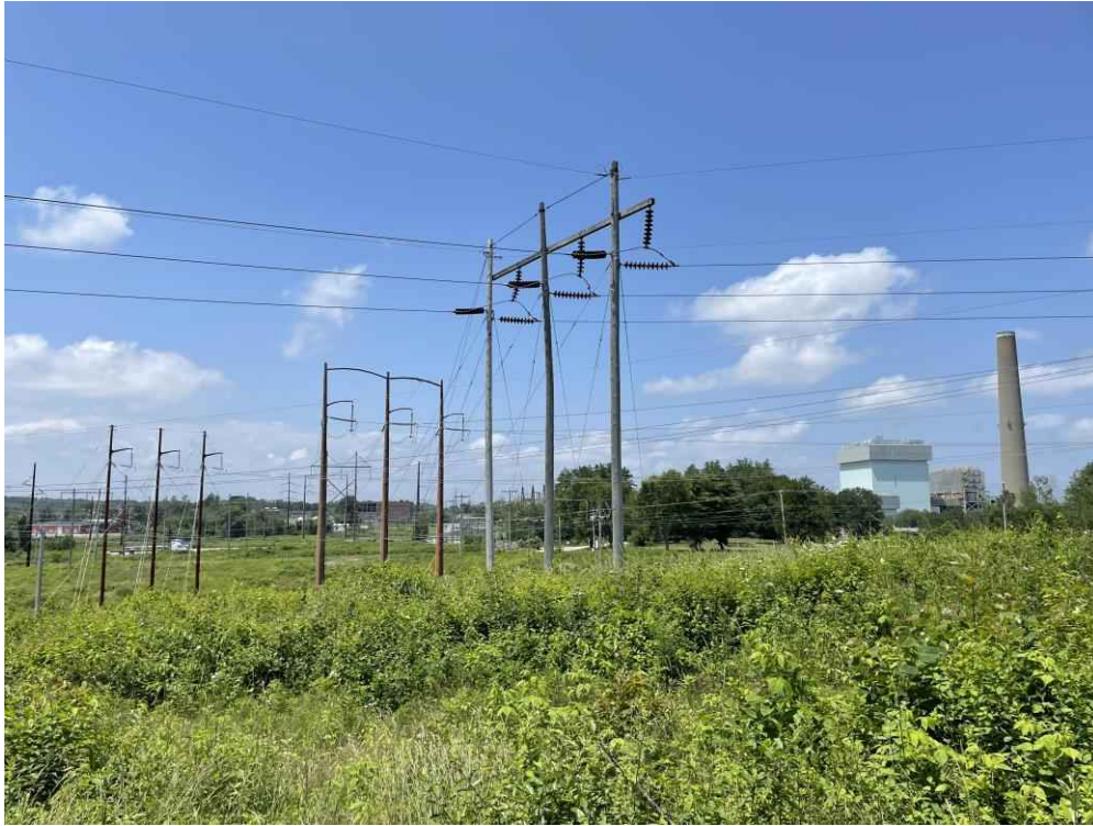
Photograph No. 23: Looking northwest near Wetland PW-3 (PEM1/PSS1E) between Structures 1 and 2 on the T13 Line ROW off Gosling Road, Portsmouth, NH.
