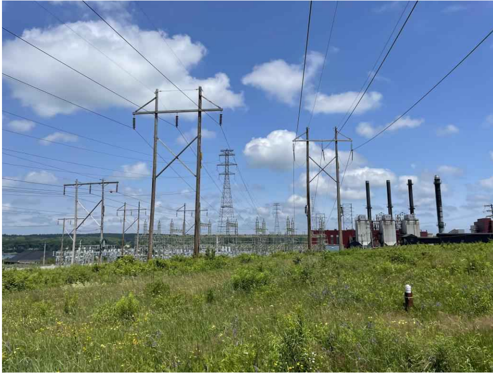
Photograph No. 21: Looking northeast at Structure 1 on the T13 Line ROW off Gosling Road, Portsmouth, NH.
