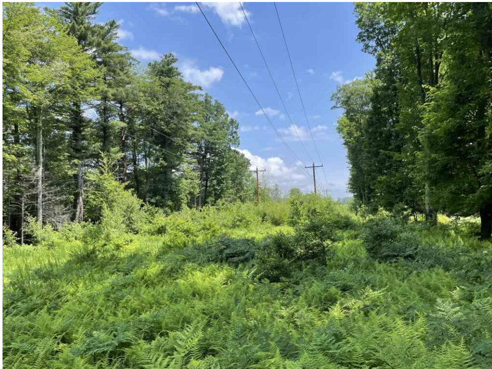
Photograph No. 10: Looking north towards Structure 86 on the 3171 Line ROW off Ocean Road, Portsmouth, NH.
